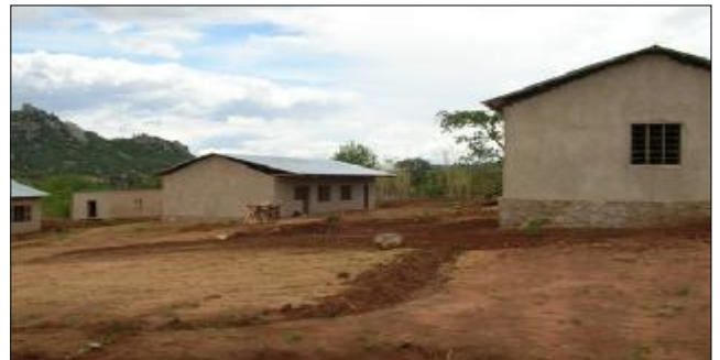
Construction is nearly complete on most of the buildings at the Tanzanian orphanage.
