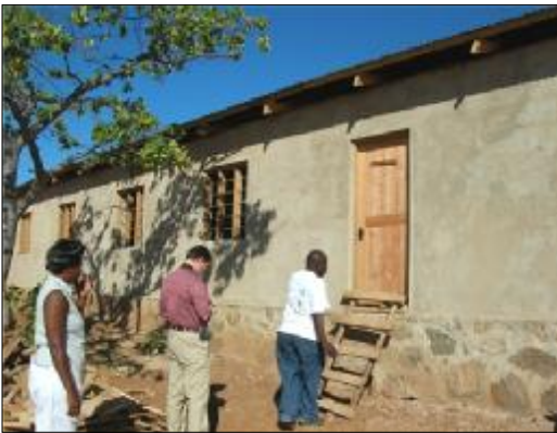
Mpeli and Neema Mwaishumbe give Kip Miller, center, a tour of the orphanage's newly constructed dormitory.
