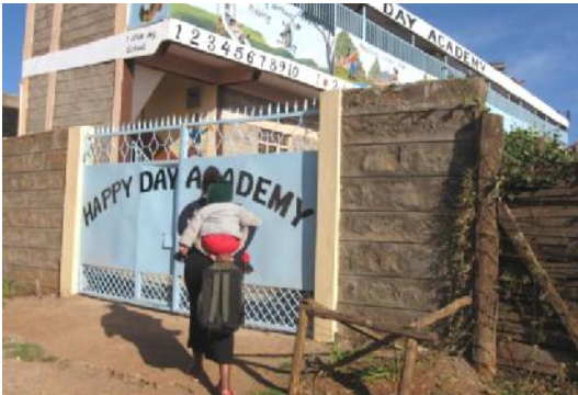
With construction complete, additional classrooms are now available allowing more children to come to school.
