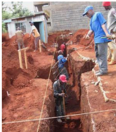
The foundation is being laid for the new Koinonia Church building.
